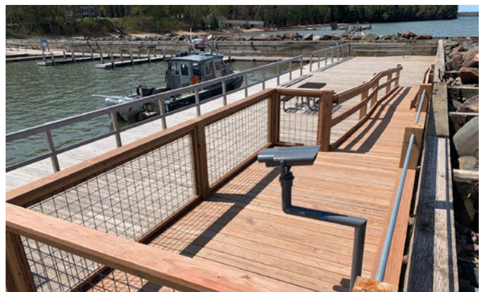
Accessible viewing platform up to binocular on a dock at Little Sand Bay. Credit: National Park Service
